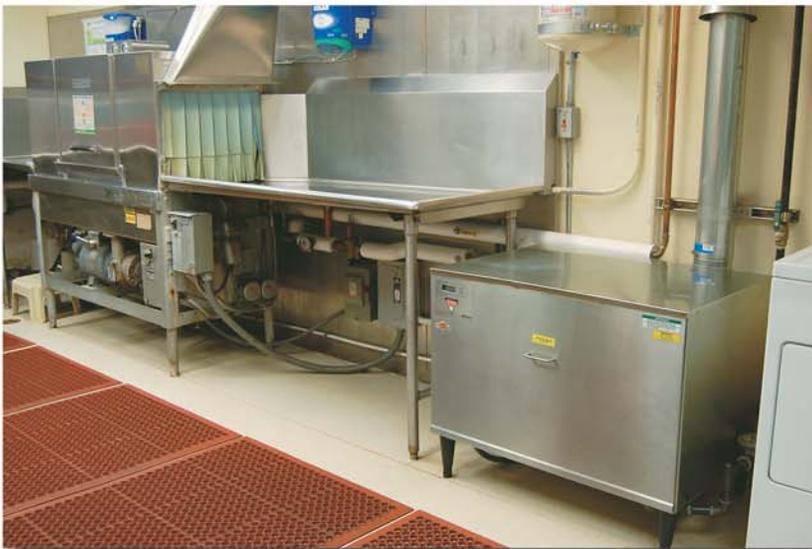
**Oregon's Salem-Keizer Public Schools replaced costly to operate electric boosters with compact, energy-efficient Vanguard PowerMax™ 200 gas booster heaters (shown at right) that reliably provide 180°F sterilizing rinse water to the kitchens' dishmachines.**
