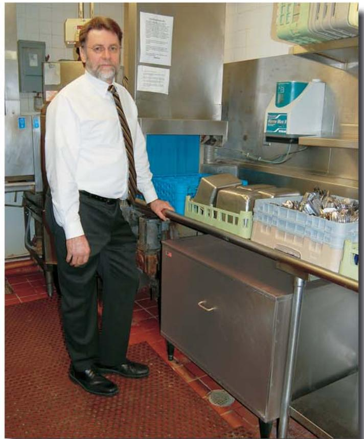
**Ric Holderbaum, of The Dussin Group, says Vanguard's compact PowerMax™ 200 Gas Booster Heaters (shown under dish table) reliably provide the 180°F sterilizing rinse water for The Old Spaghetti Factory's dishmachines.**
